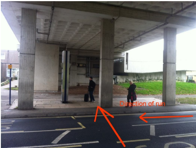
FINISH Central concrete pillar
