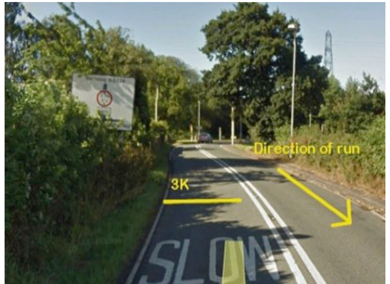
3K Approaching sharp left bend. Midway between Height restriction sign and "slow" sign on road
